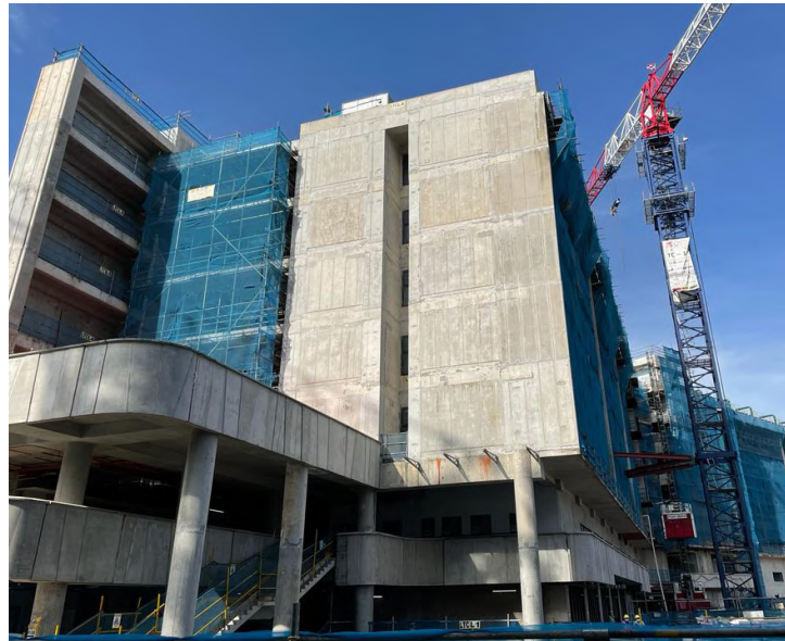
Ren Ci @ Woodlands under construction, taken during the topping out ceremony
