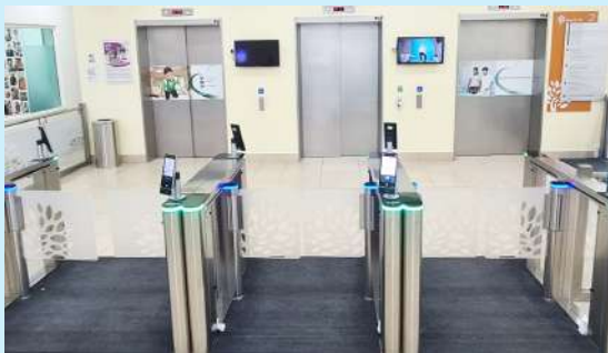
Automated gantry system at Ren Ci Community Hospital
